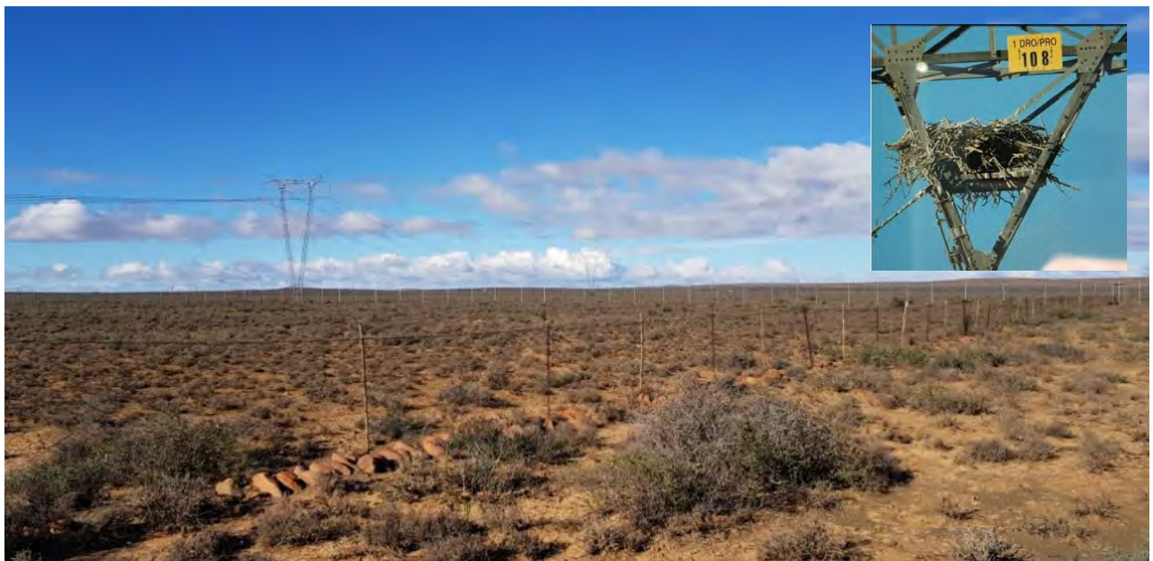
Figure 2: The Droërvier Proteus 400kV HV line that runs through the study area. The insert shows the Martial Eagle nest on Tower 108.
