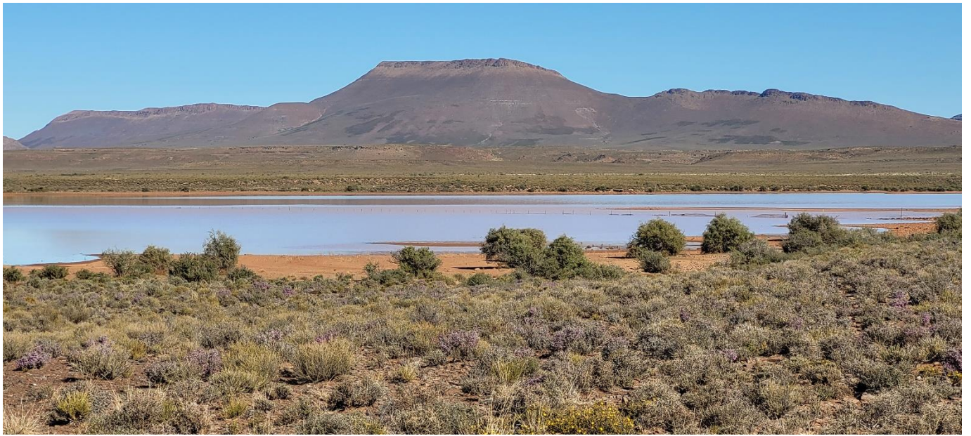
Figure 3: Ground dam – Focal Point 2
