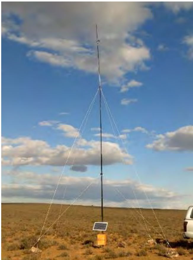
Figure 4: Short mast monitoring system set up
