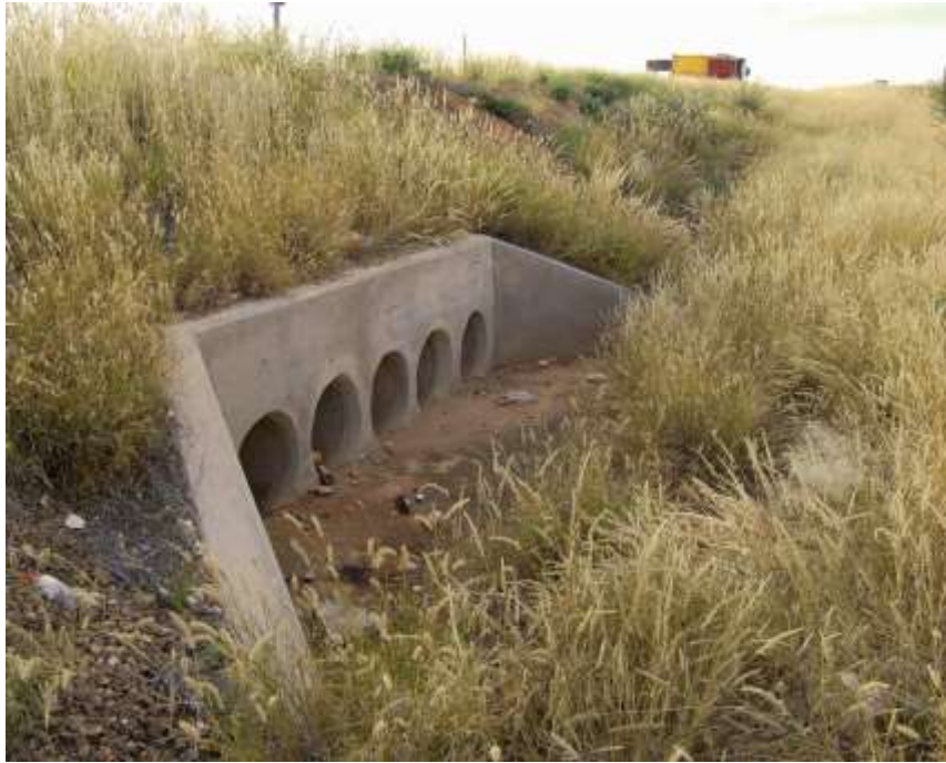
Figure 17 Culvert
