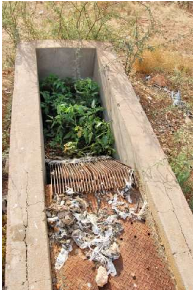
Figure 12 Intake structure
