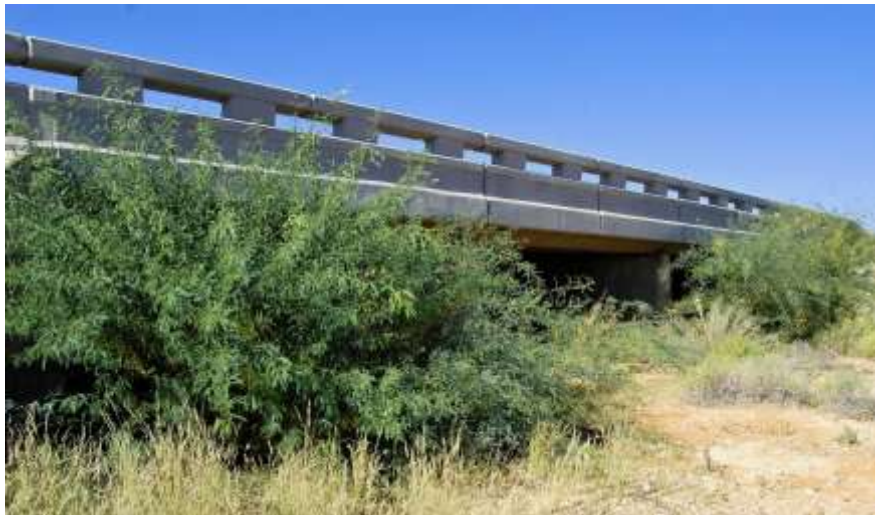
Figure 8 N10 road bridge
