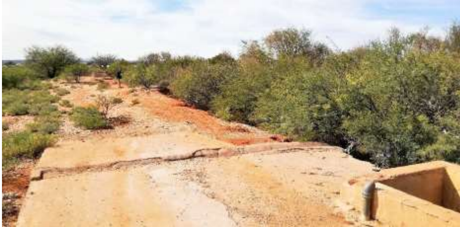
Figure 9 WWTWs Intake (Photo Clinton Geysler)
