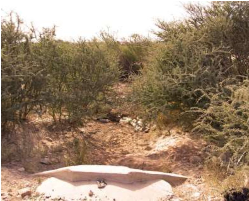
Figure 20 Downstream from culvert
