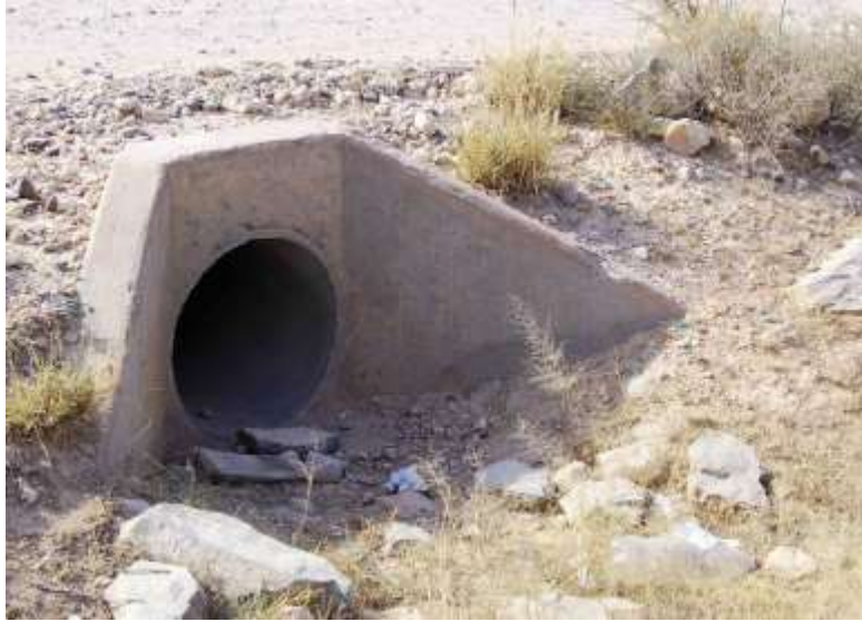
Figure 19 Culvert of longer drainage line
