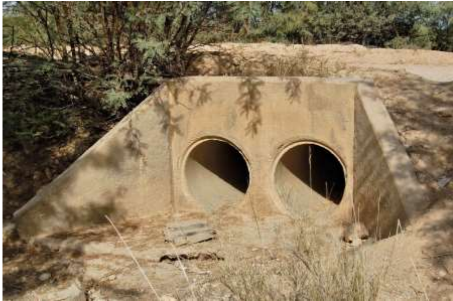
Figure 17 Culvert downstream of sewage pump station
