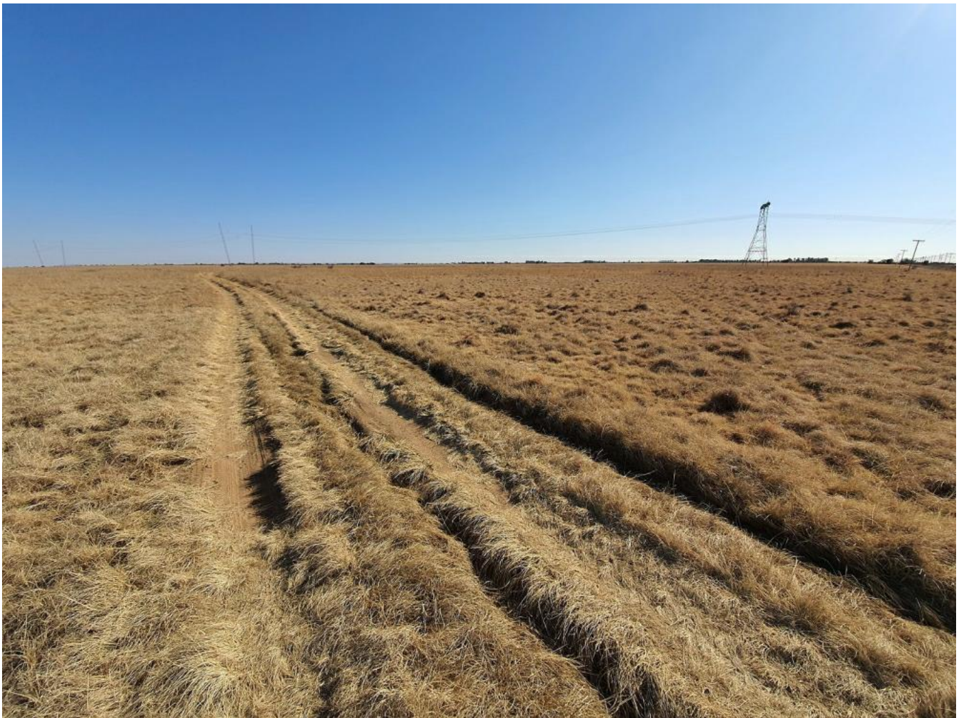
Figure 2: High voltage lines in the application site.
