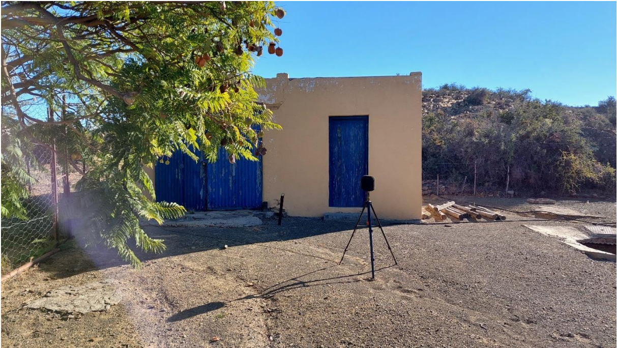
Photos B.2: Measurement location at SGEKLTSL02
