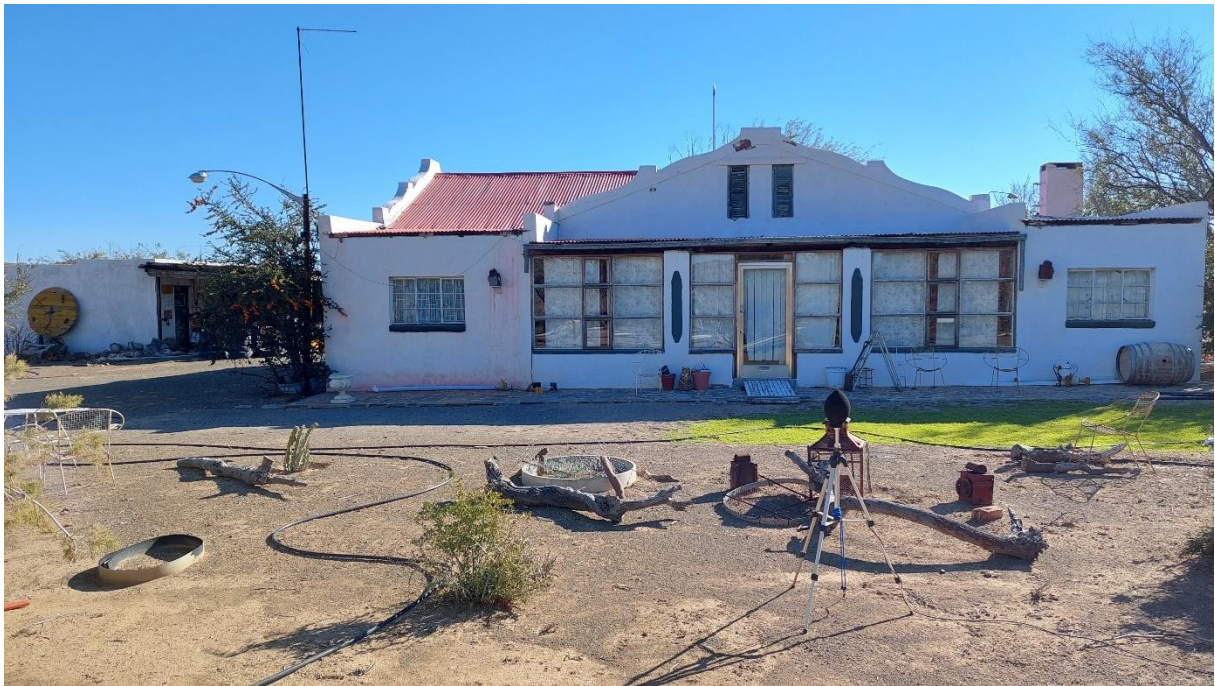
Photos B.1: Measurement location at SGEKLTSL01
