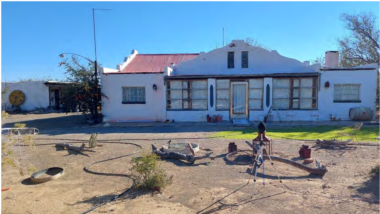
Photos B.1: Measurement location at SGEKLTSL01
