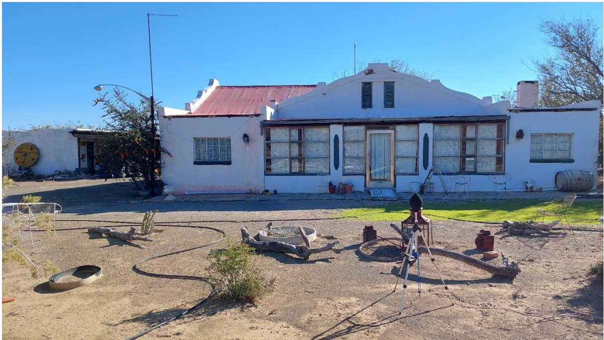
Photos B.1: Measurement location at SGEKLTSL01
