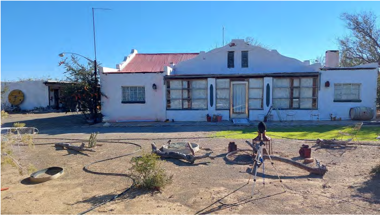
Photos B.1: Measurement location at SGEKLTSL01
