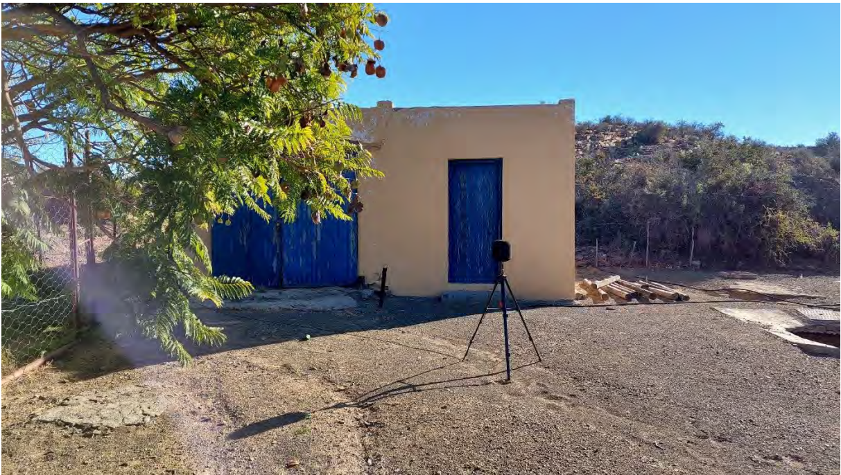
Photos B.2: Measurement location at SGEKLTSL02
