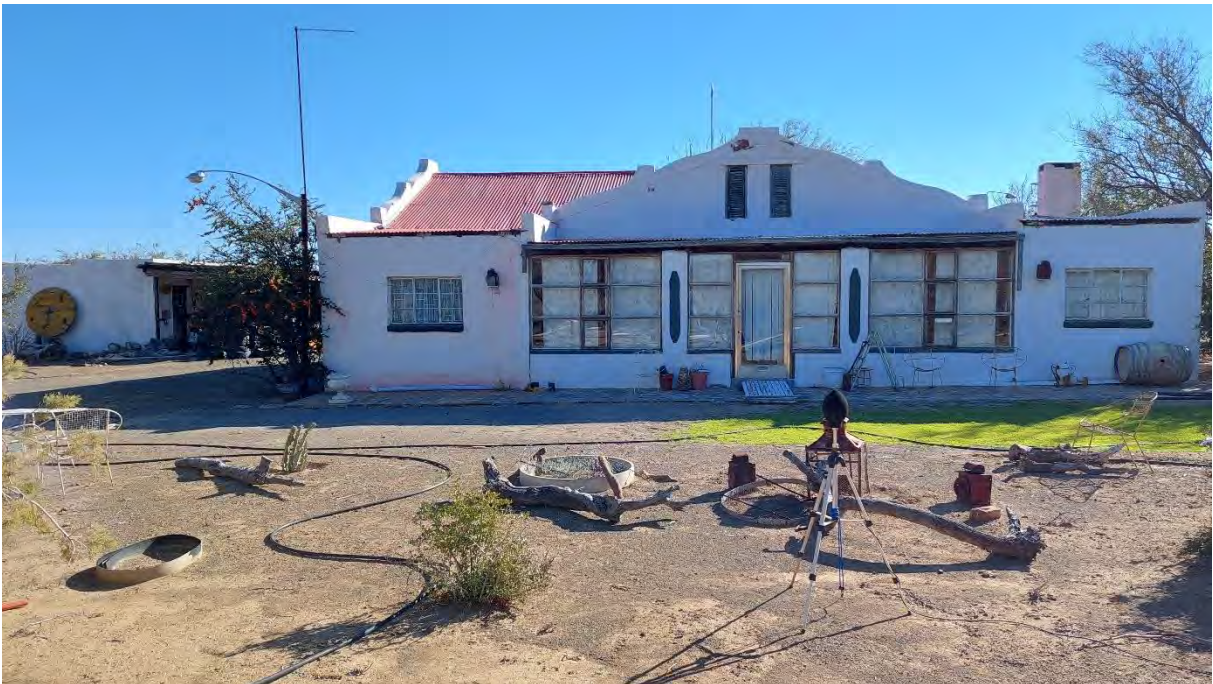
Photos B.1: Measurement location at SGEKLTSL01
