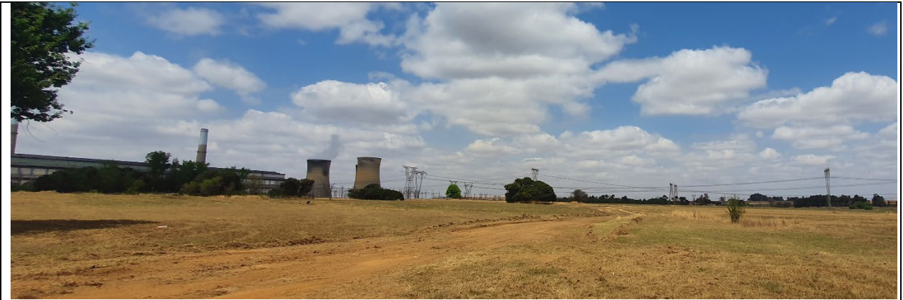
Viewpoint 1: Pullens Hope Road - looking south. The 132 kV powerline will be visible, but obscured and assimilated by the existing powerlines.
