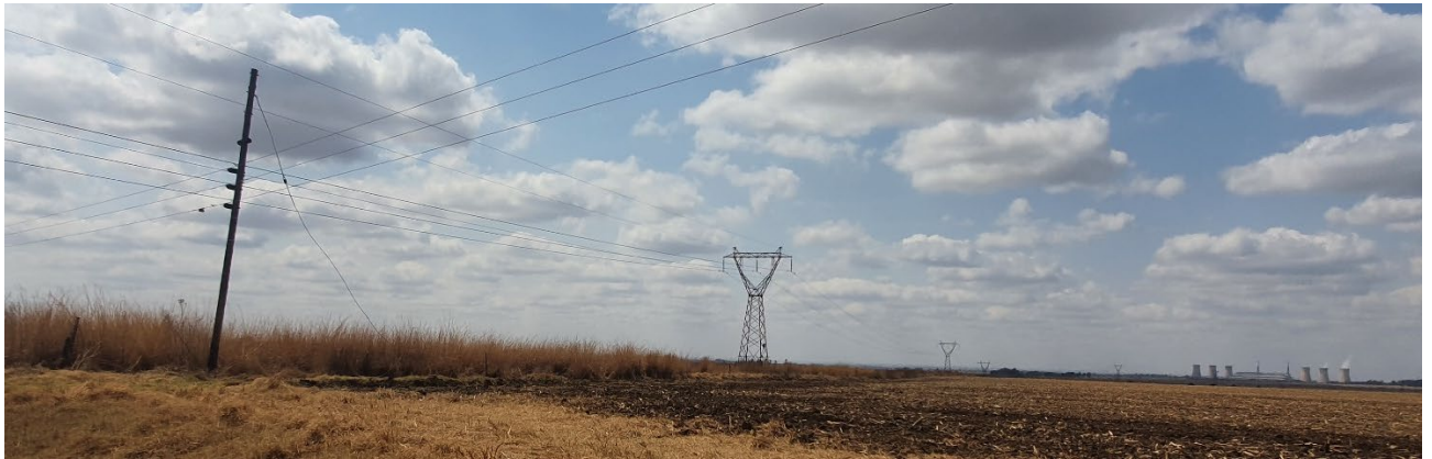
Figure 5-6: Existing Eskom Hendrina-Abina 132 kV powerline
