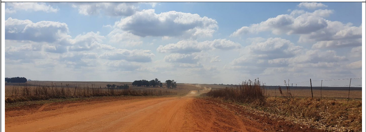
Viewpoint 15: Hendrina WEF Substation– looking north-west. Powerline Alternative 1 and 2 will be routed adjacent to this gravel road and will be highly visible to receptors (right side of the photograph) in the foreground. The substation will be located on the farm on the left (west) and will be visible in the foreground.
