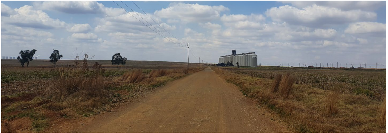
Figure 5-5: Afagri grain silo
