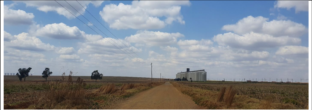
Viewpoint 8: Afgri grain silo – looking east toward Powerline Alternative 1 routed in front of the grain silo. The powerline will be highly visible in the foreground.
