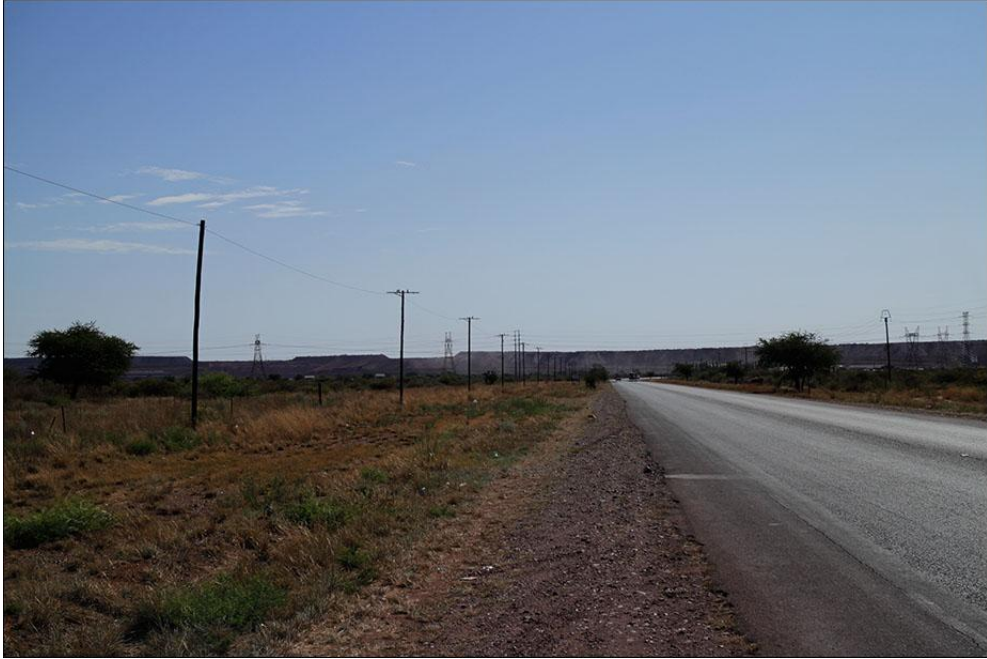
Photo 10: Gravel road shoulders
