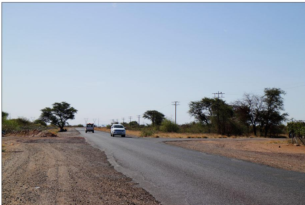
Photo 7: Current intersection as seen from the south
