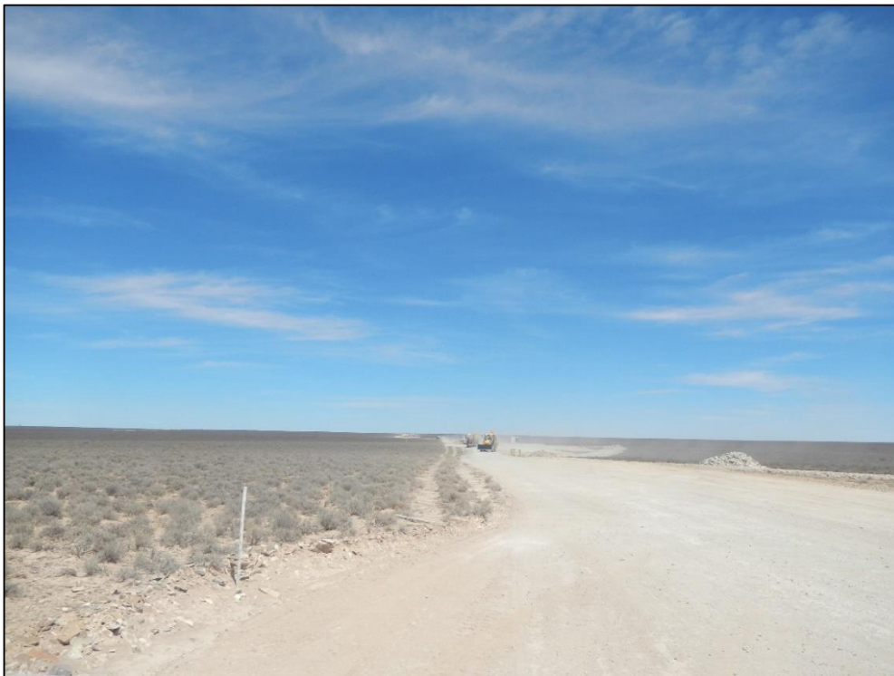
Figure 22: View of the construction activities associated with the proposed Khobab Wind Farm. During the time of the in-field investigation it was noted that this wind farm was still in the early stages of construction and no turbines had thus been erected.
