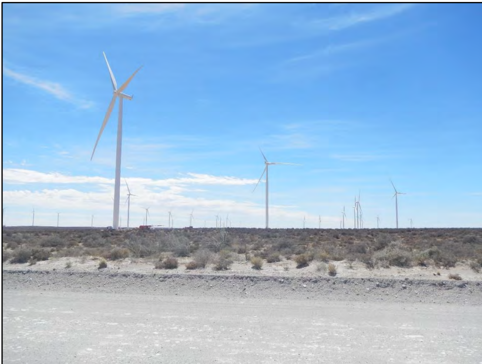
Figure 19: Wind turbines at Loerisfontein Wind Farm
