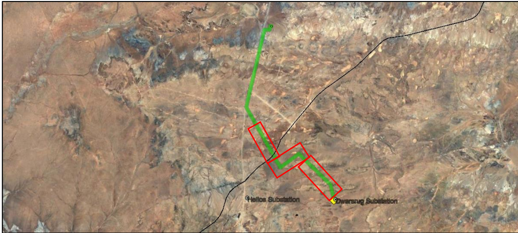
Figure 2: View of the proposed corridor for the new power line to link the Loeriesfontein Substation and the Dwarsrug Substation. The areas blocked in red indicate the low hills and drainage lines that are considered to be sensitive.
