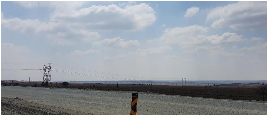
Figure 5-4: Existing 132 kV powerline extending across the site and over the R76. Photo taken at VP3 looking toward the project.
