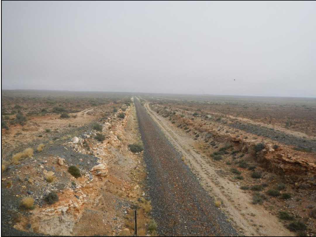
Figure 18: View of the remnants of an old railway line which traverses the northern section of the application site. Note that no railway tracks are present.
