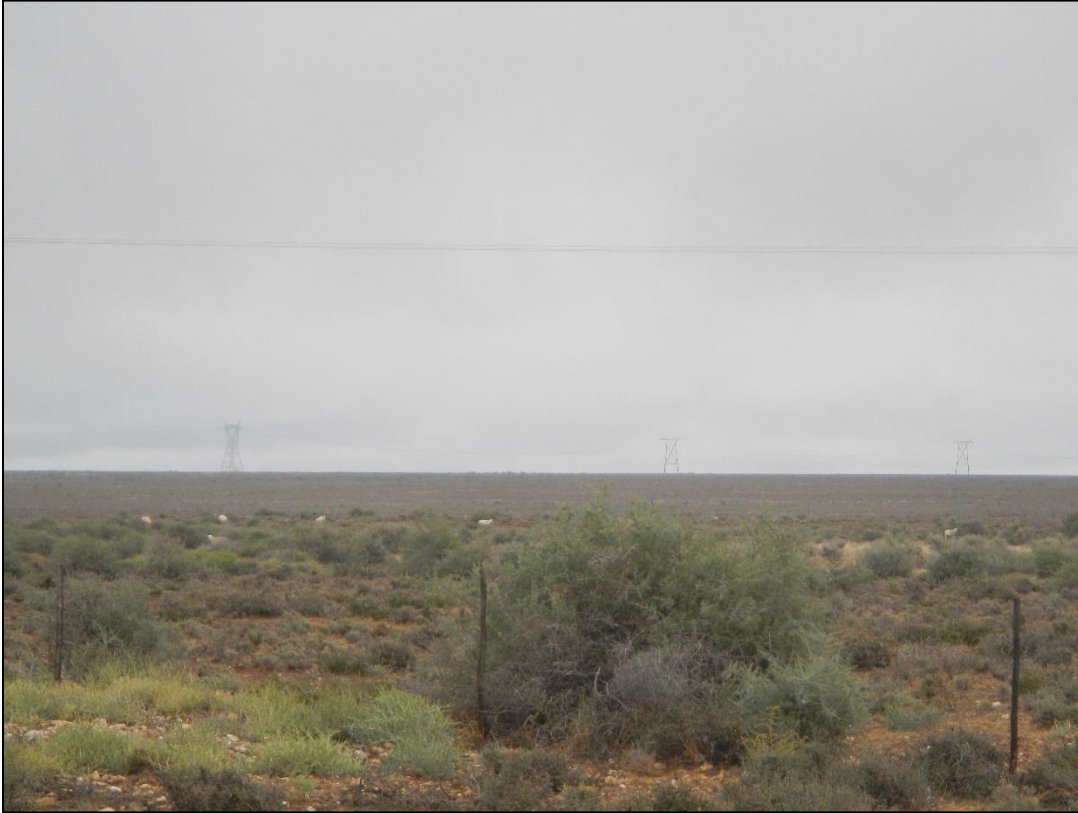
Figure 37: Typical view of the existing high voltage power lines that can be found to the south-west of the farmstead / residential dwelling at VR 4.
