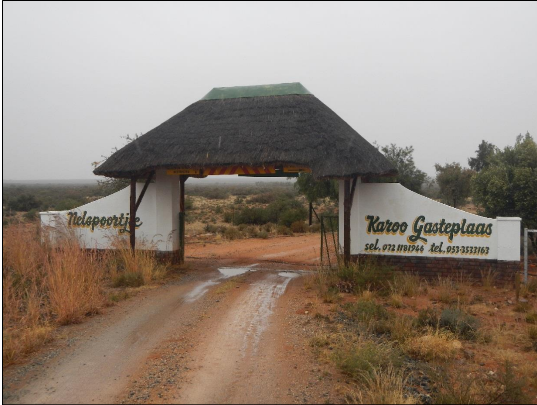
Figure 23: View of the entrance of the Nelspoortjie Karoo Guest Farm (VR 2) which is accessible via the R357 Copperton Road
