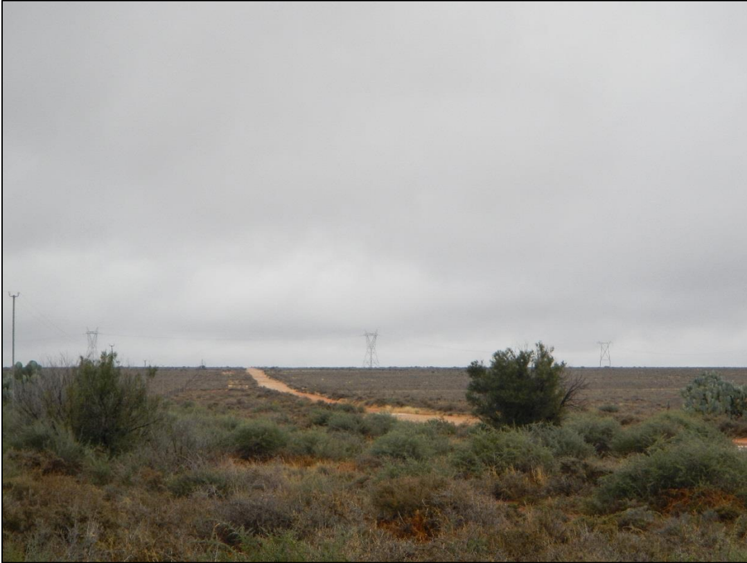
Figure 43: View of the existing high voltage power line which can be found to the south-west of the farmstead / residential dwelling at VR 11. This power line is expected to alter the natural / scenic character of the surrounding area slightly and lessen the visual contrast of the proposed Aletta Wind Energy Facility.
