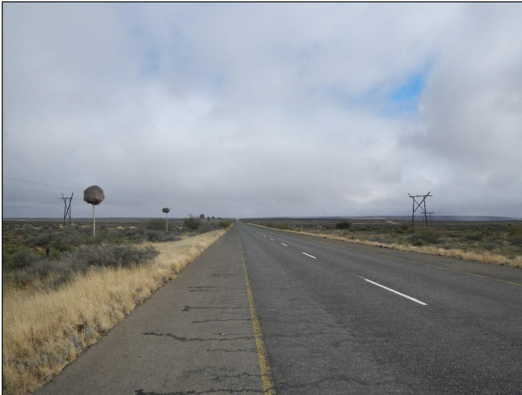
Figure 30: Photo of existing high voltage power lines which traverses a section of the R357 tar road.
