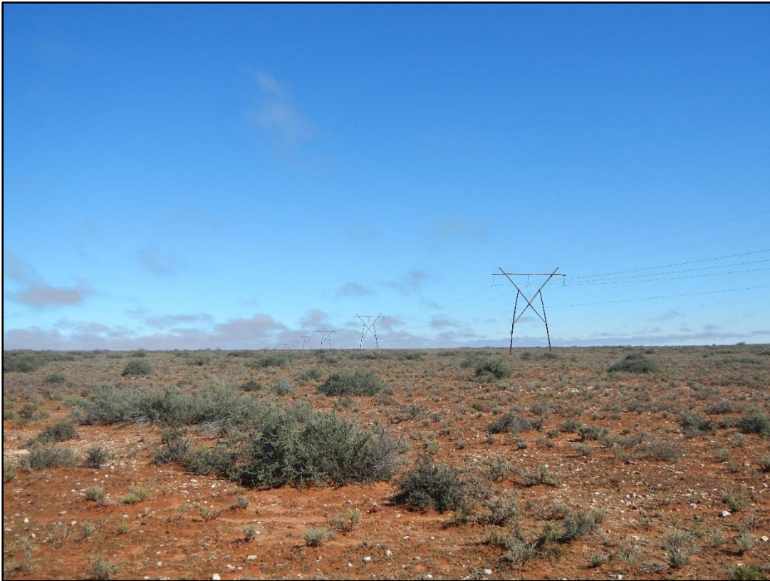
Figure 17: View of the existing high voltage power lines found within the study area which are expected to alter the overall natural / scenic character of the study area slightly and lower the visual contrast associated with the proposed wind energy facility.
