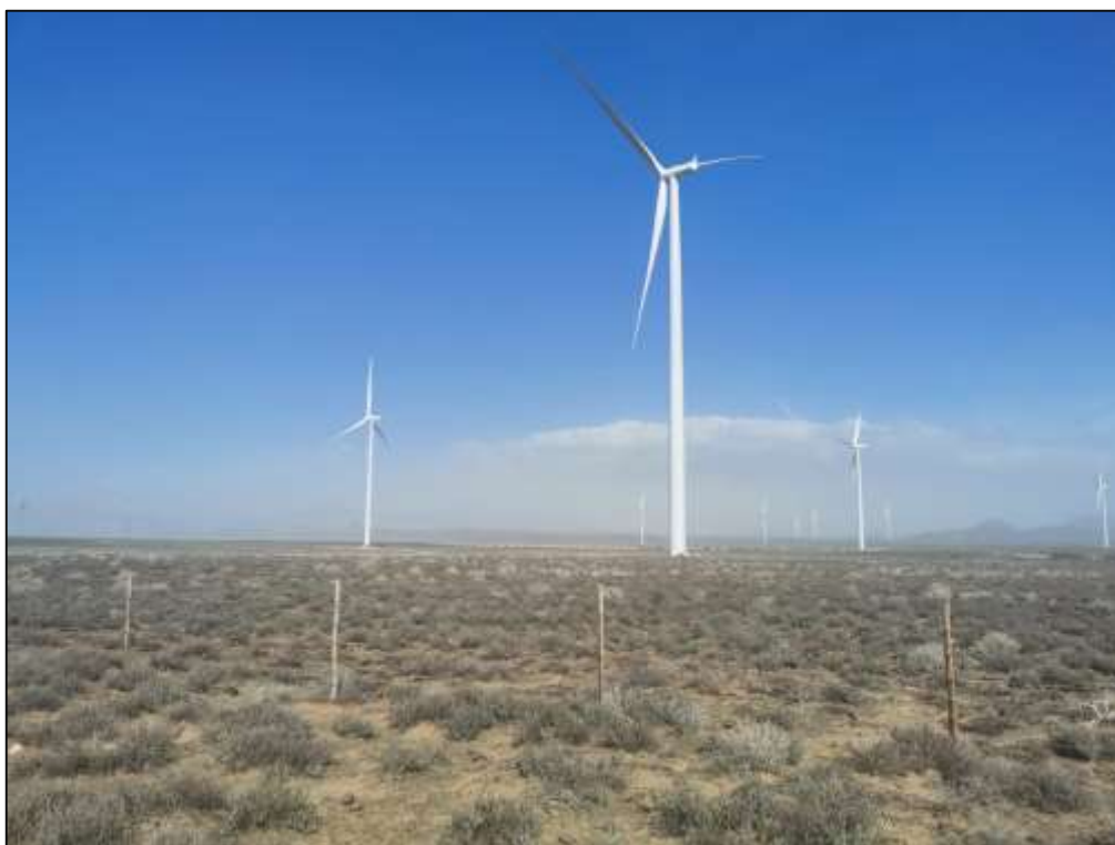
Figure 23: Operational wind turbines at Perdekraal East Wind Farm
