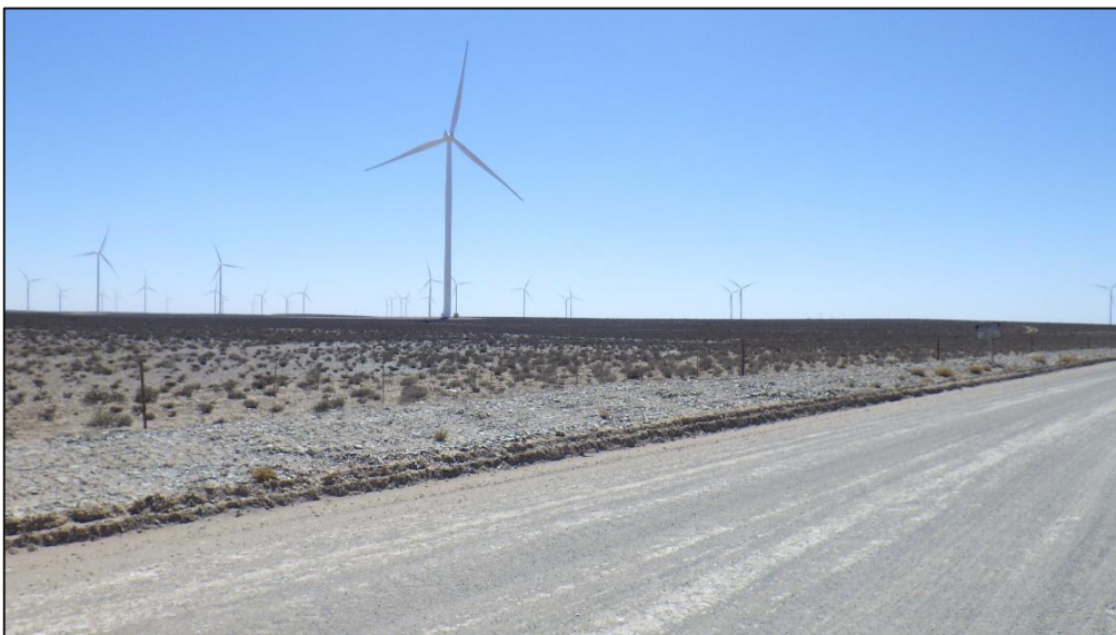
Figure 20: Operational wind turbines at Loeriesfontein 2 Wind Farm
