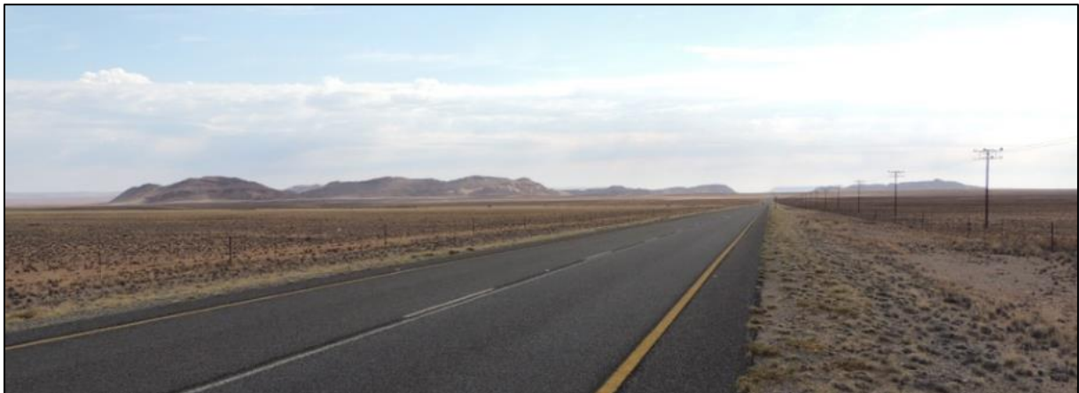
Figure 5: Photograph of the N14 National Road northbound just before Aggeneys town.
