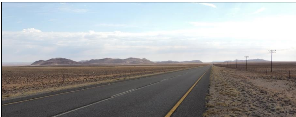
Figure 5: Photograph of the N14 National Road northbound just before Aggeneys town.
