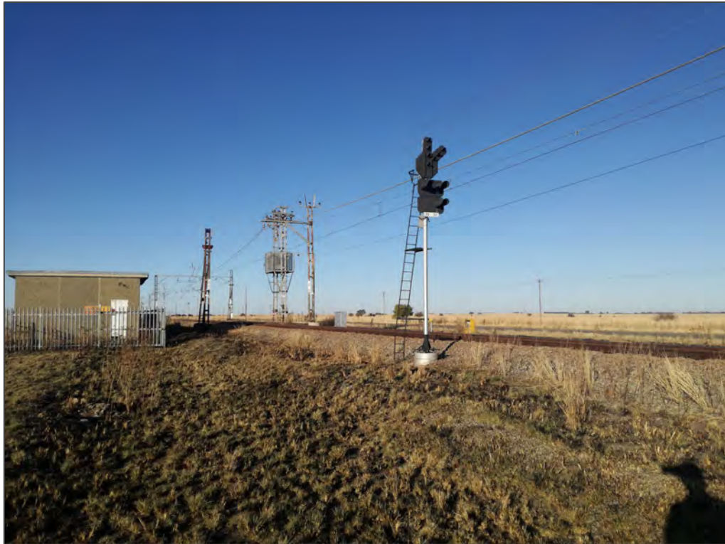
Figure 11: Railway infrastructure adjacent to the R502 Main Road
