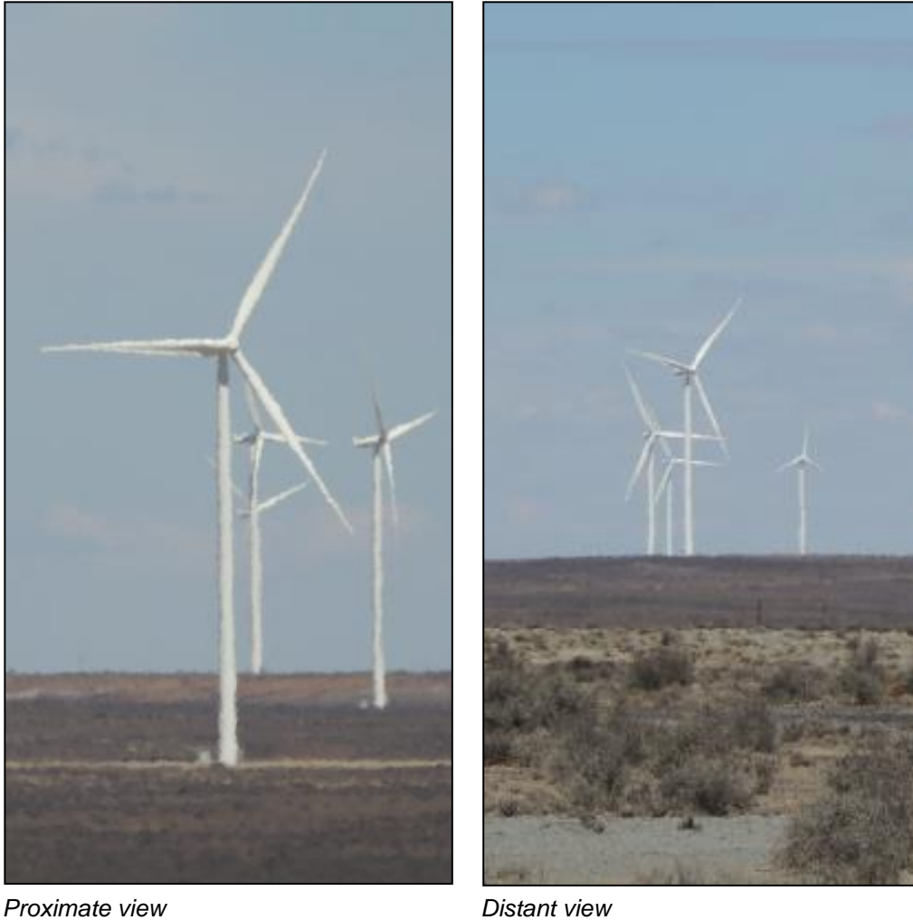
Figure 20: Photographic material used to inform the photomontages was based on photographs of the existing Khobab & Loeriesfontein wind farms as they reflect similar landscape conditions.
