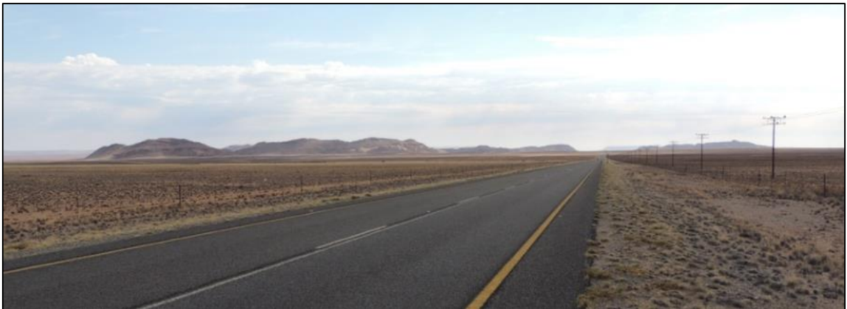
Figure 6: Photograph of the N14 National Road northbound just before Aggeneys town.
