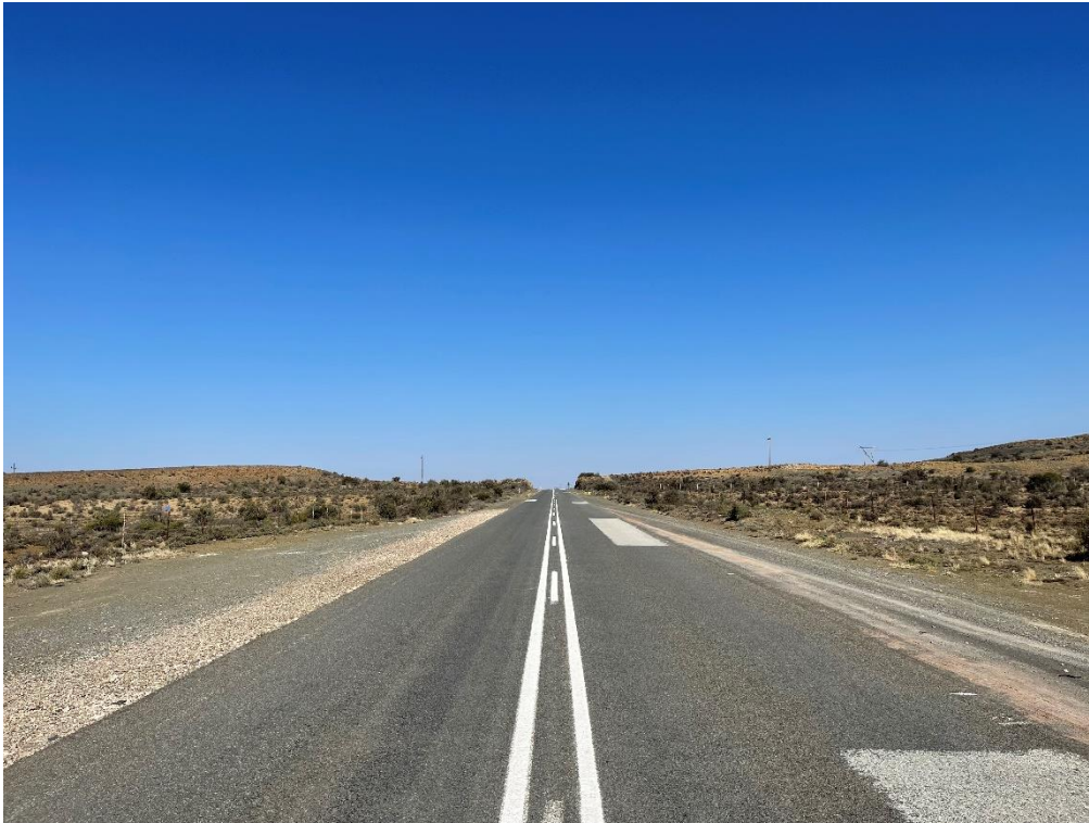
Figure 7.7 Existing Access to Koup 2 - South approaching
