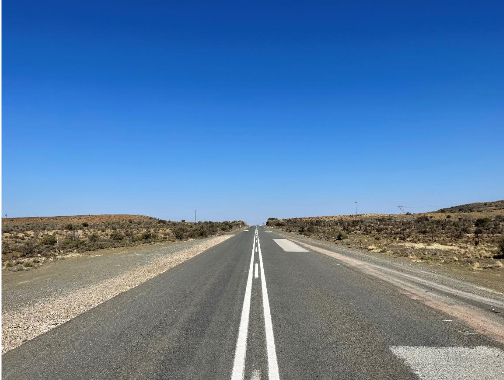
Figure 7.7 Existing Access to Koup 1 - South approaching
