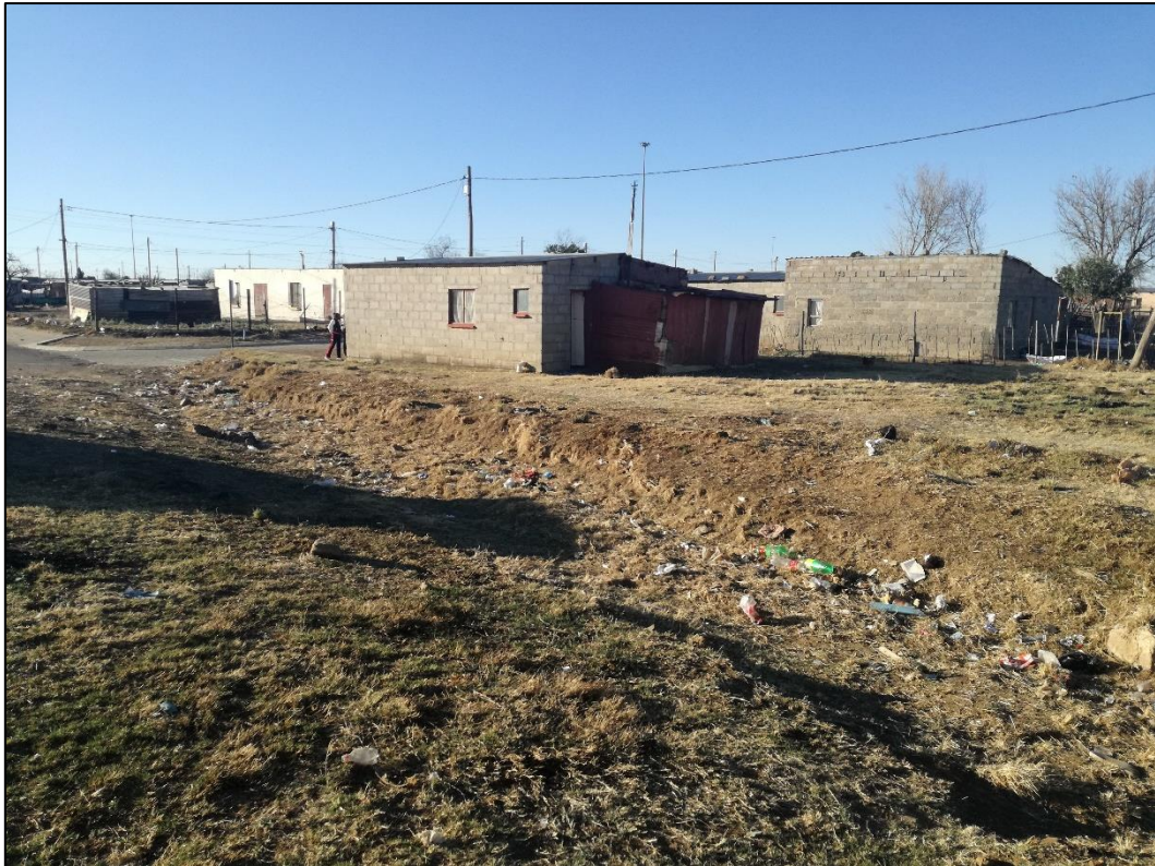
Figure 18: Urban and infrastructural built form of Kgakala Township
