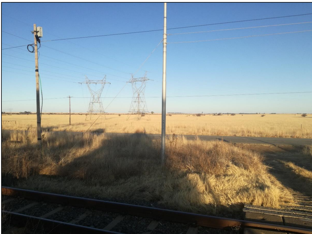
Figure 15: High voltage power lines in the study area
