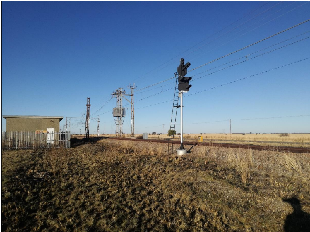
Figure 12: Railway infrastructure adjacent to the R502 Main Road
