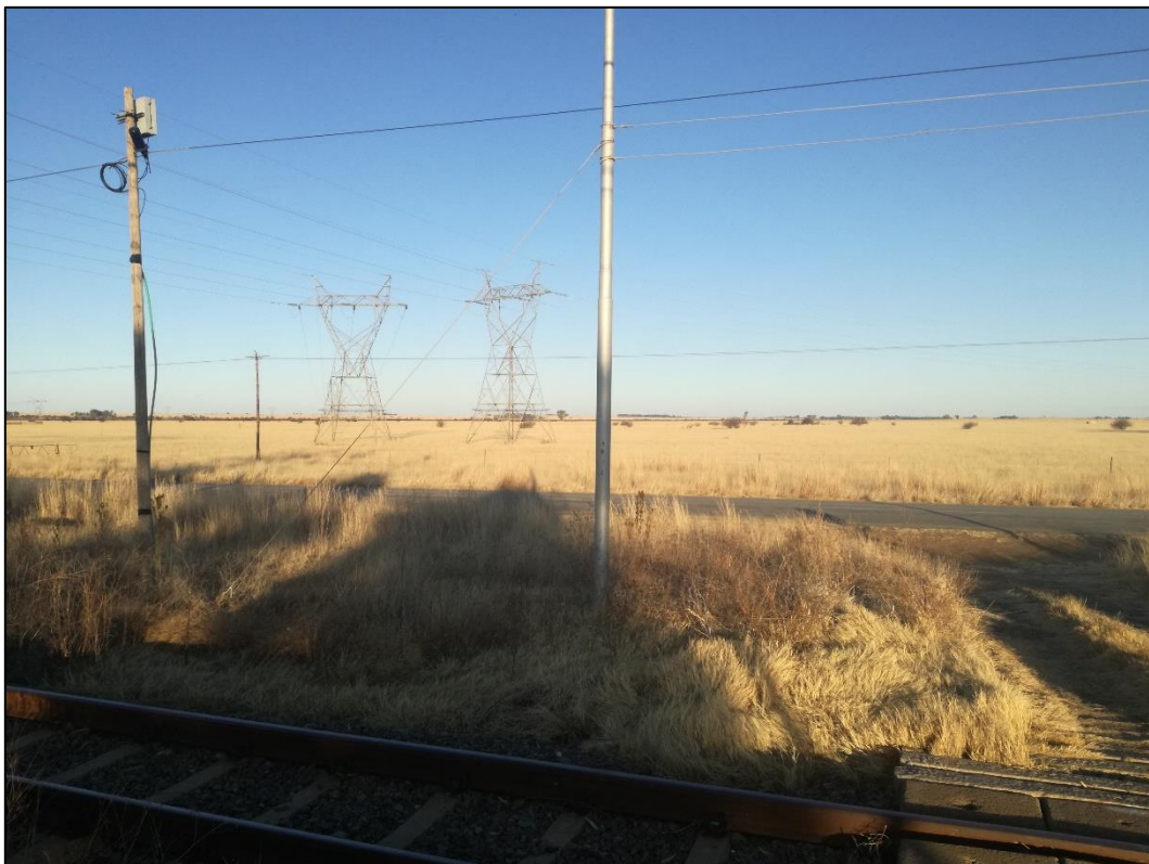
Figure 13: High voltage power lines in the study area
