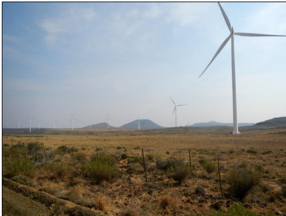
Figure 31: Wind turbines at Noupport Wind Farm, near Noupport, Northern Cape Province.
