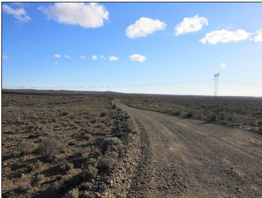
Figure 26: View of 400kV power lines to the east of the Koup 1 WEF application site.
