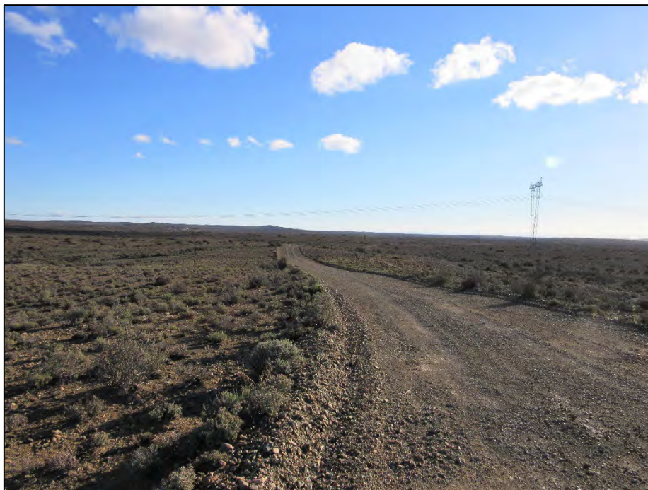
Figure 26: View of 400kV power lines to the east of the Koup 1 WEF application site.
