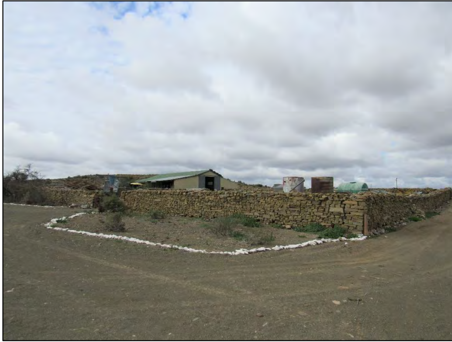
Figure 23: Farm buildings and associated infrastructure south of the Koups 2 WEF application site.
