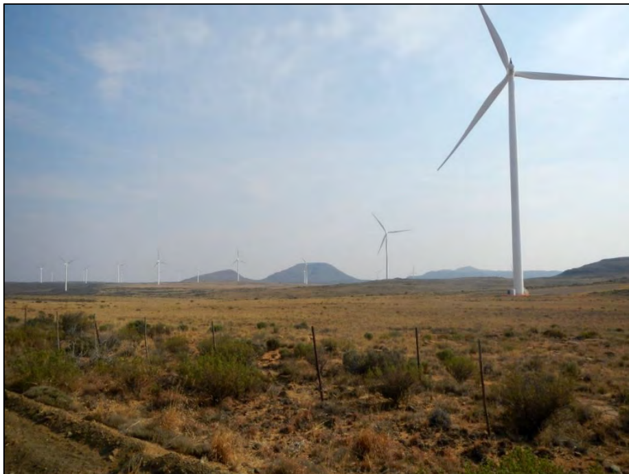
Figure 31: Wind turbines at Noupoort Wind Farm, near Noupoort, Northern Cape Province.
