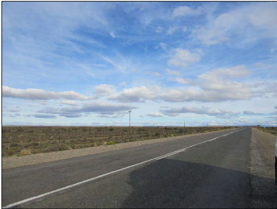
Figure 24: View southwards along the N12 National Route on the eastern boundary of Koup 2 WEF study area.
