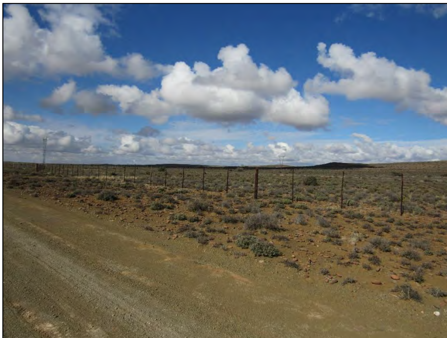
Figure 26: Distant view of 400kV power lines to the east of the Koups 2 WEF application site.
