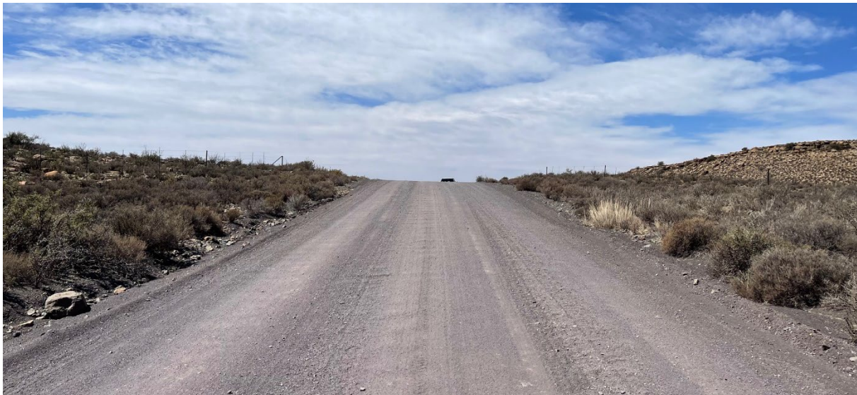
Figure 7.9 Vertical Curve at Km 89.55 on Road DR2312 with a vehicle in the background
