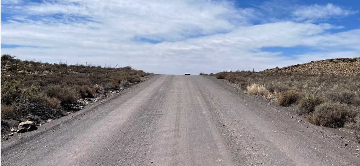
Figure 7.10 Vertical Curve at Km 89.55 on Road DR2312 with a vehicle in the background
