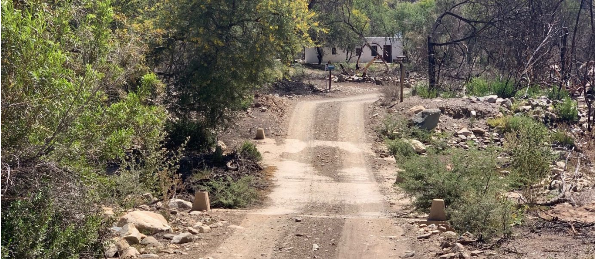
Figure 14:4 Typical Low-Level Concrete structure
