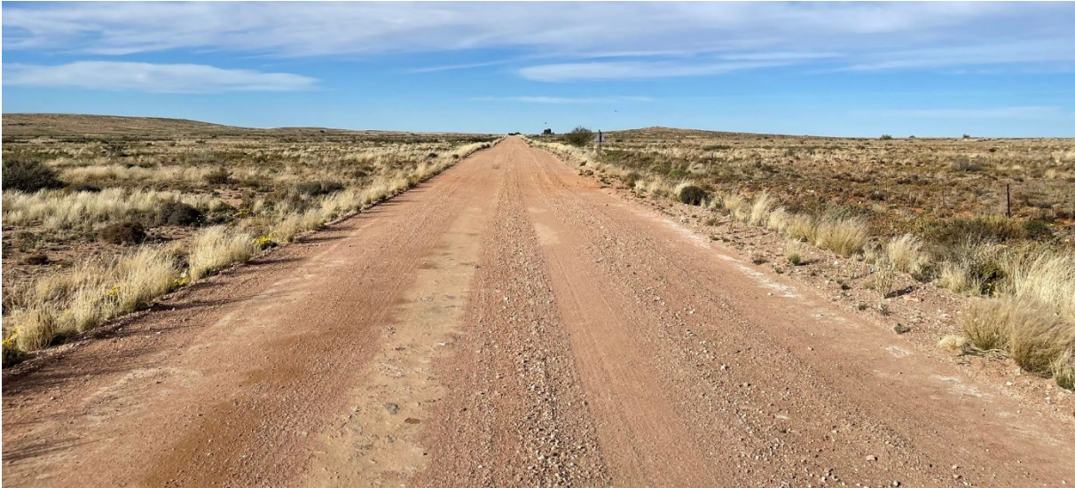
Figure 7.14 Existing Road DR2986 @ Km 148.11 – West Approaching
