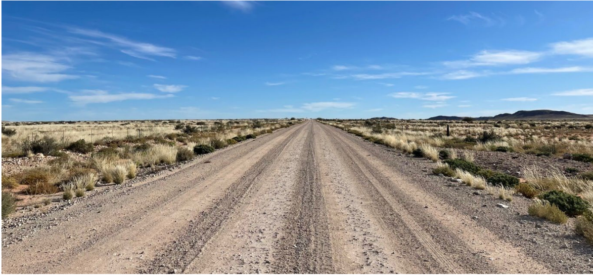
Figure 7.8 Existing Road DR2986 @ Km 153.99 – West Approaching
