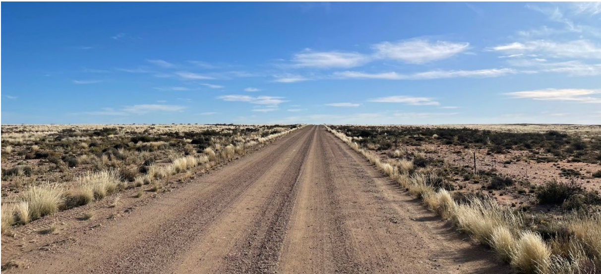
Figure 7.18 Existing Road DR2986 @ Km 142.80 – East Approaching
