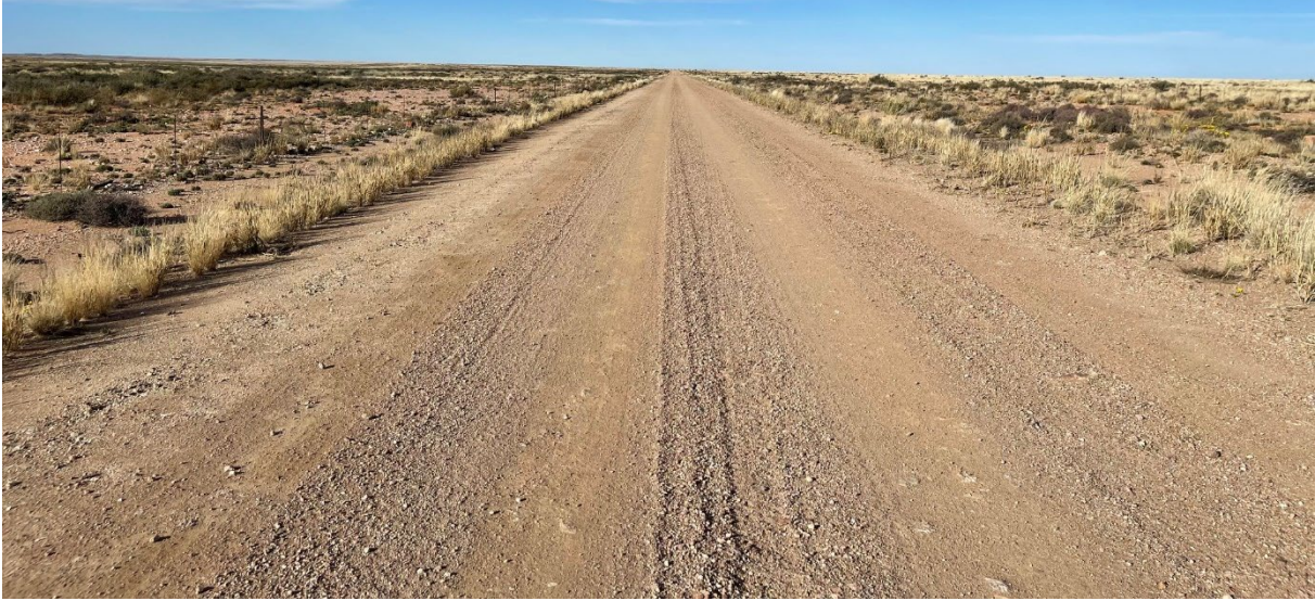
Figure 7.21 Existing Road DR2986 @ Km 142.80 – West Approaching
