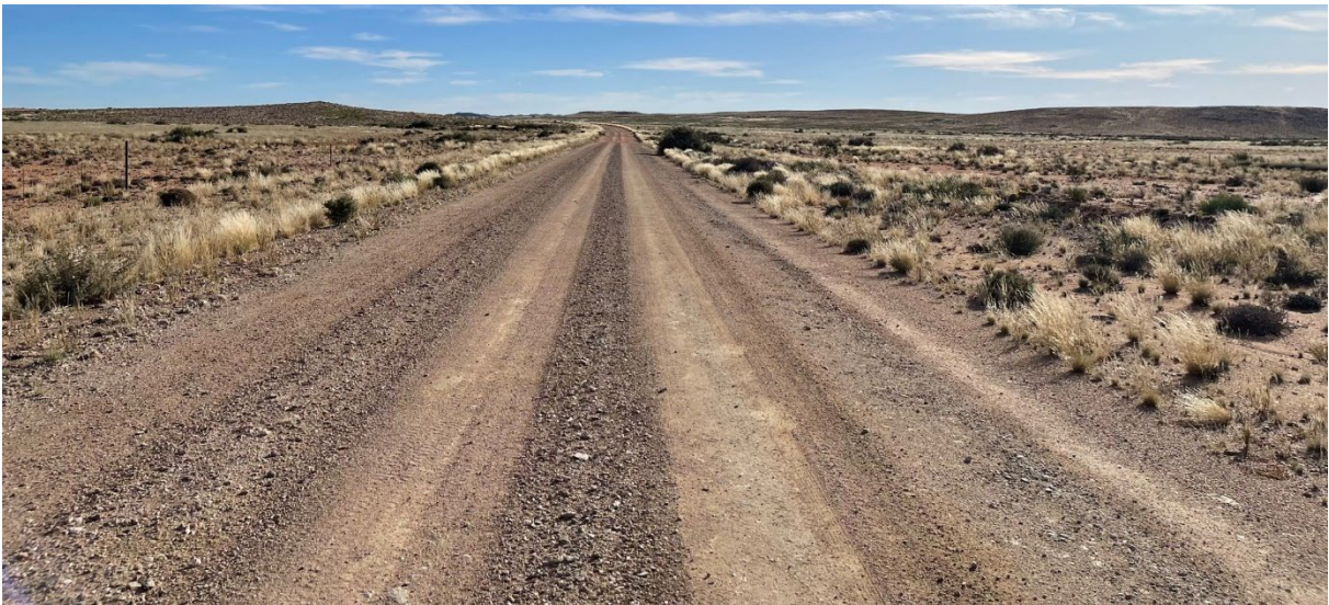
Figure 7.15 Existing Road DR2986 @ Km 146.82 – West Approaching
