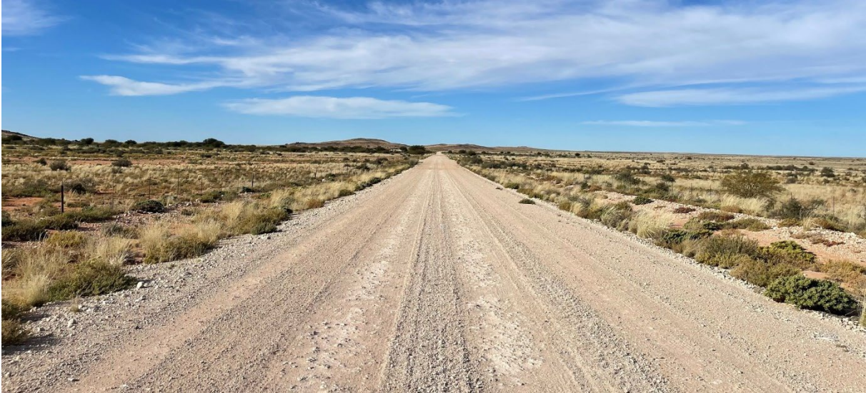
Figure 7.10 Existing Road DR2986 @ Km 153.99 – West Approaching
