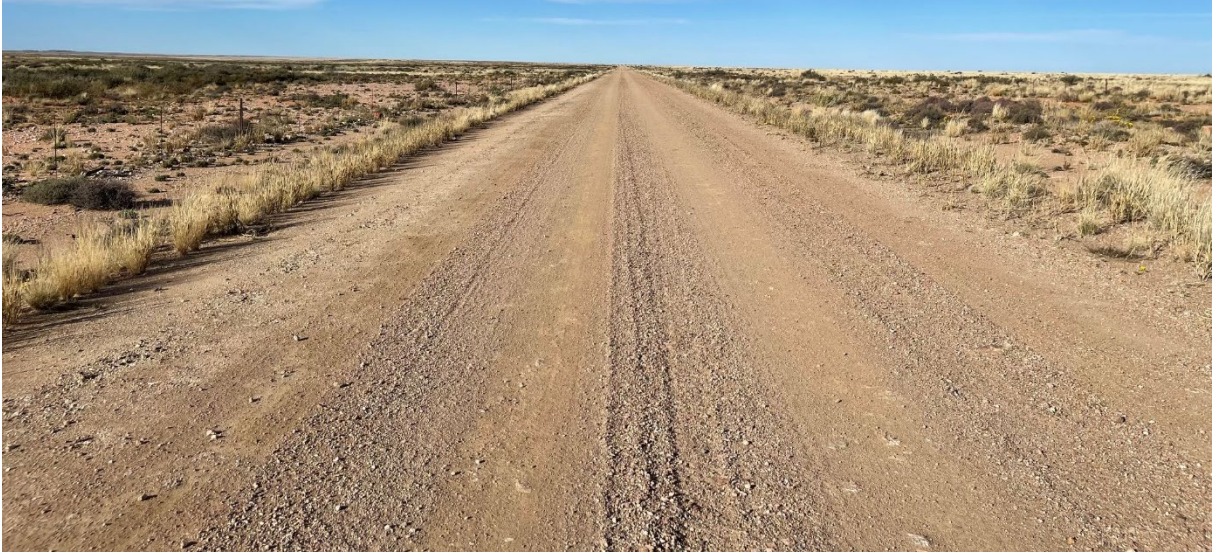
Figure 7.21 Existing Road DR2986 @ Km 142.80 – West Approaching
