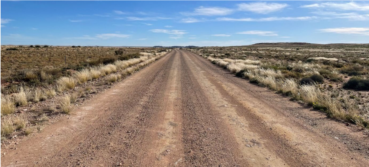
Figure 7.11 Existing Road DR2986 @ Km 148.11 – East Approaching
