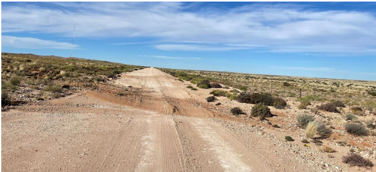
Figure 7.22 Typical erosion in drainage lines on External Roads
