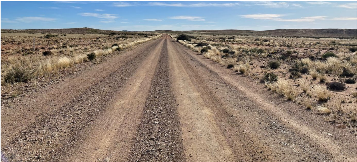
Figure 7.15 Existing Road DR2986 @ Km 146.82 – West Approaching
