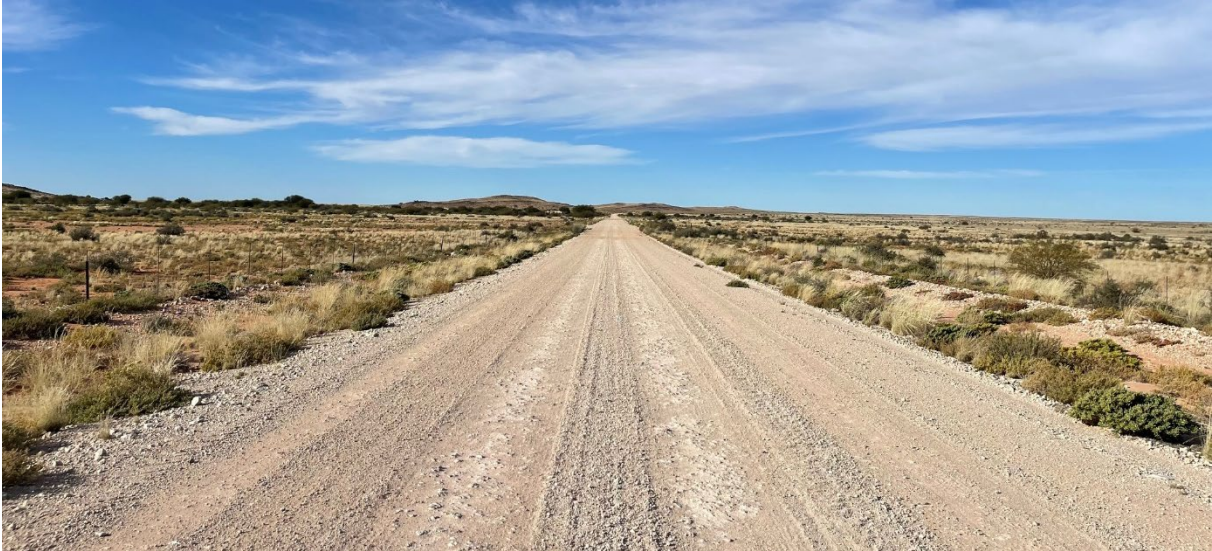
Figure 7.10 Existing Road DR2986 @ Km 153.99 – West Approaching
