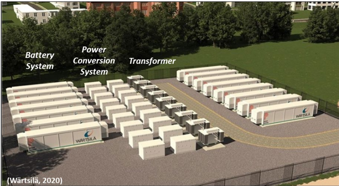
Figure 5: Pivot Power's proposed 50MW lithium-ion battery in Kemsley, Kent.
