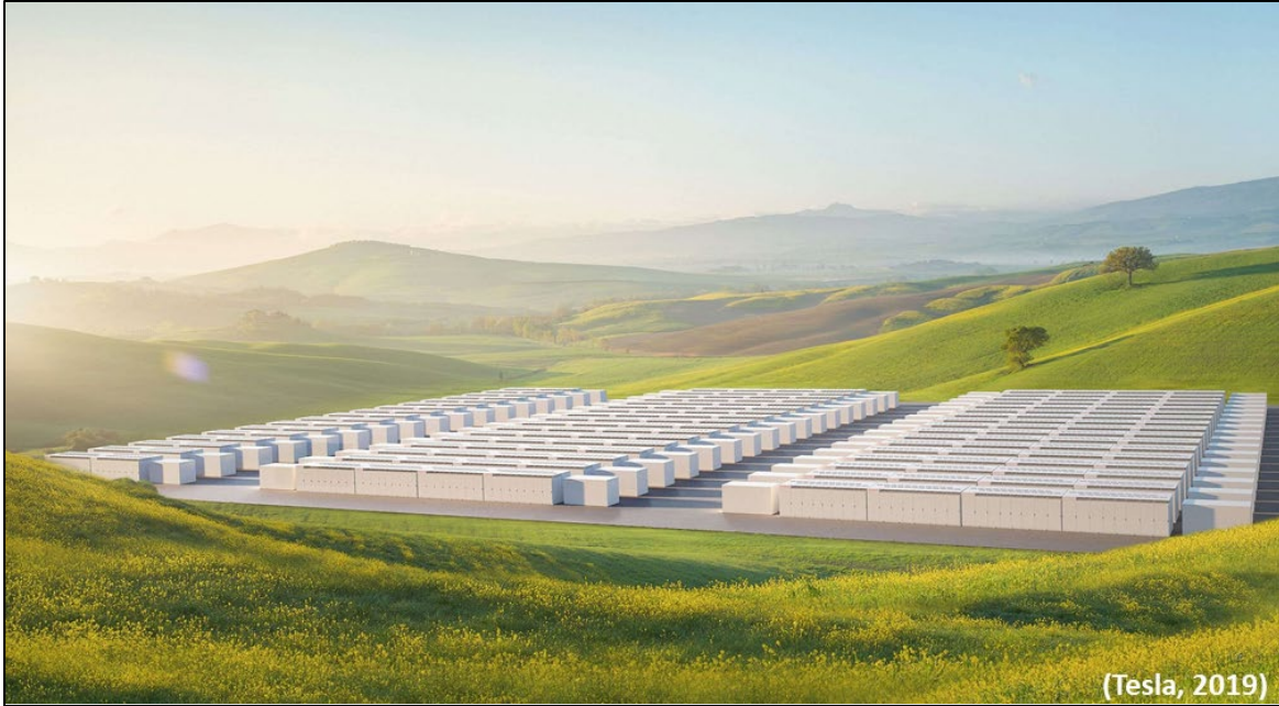
Figure 1: Tesla's Megapack Li-ion Battery (Modular System).
