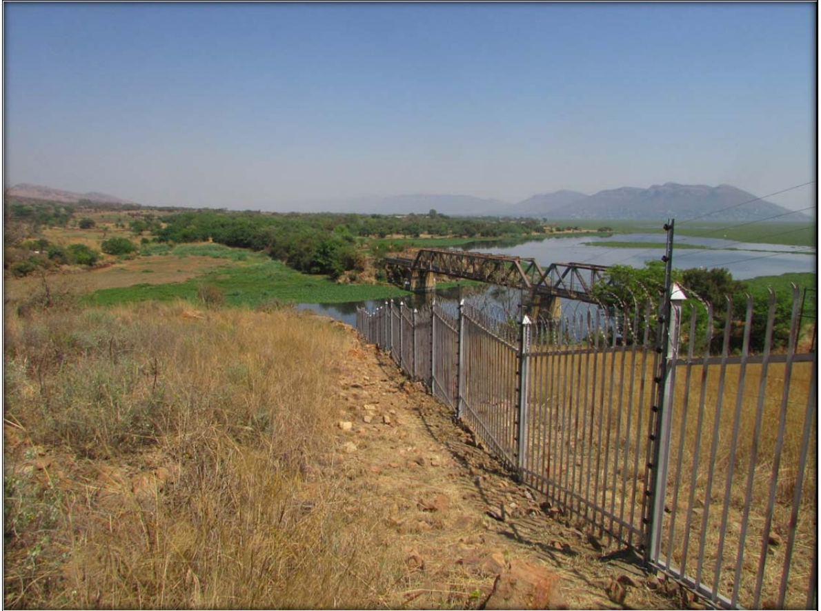
Figure 12: Estate D’Afrique boundary fence. The proposed road will link up at the bottom with an existing road at the Meerhof side.
