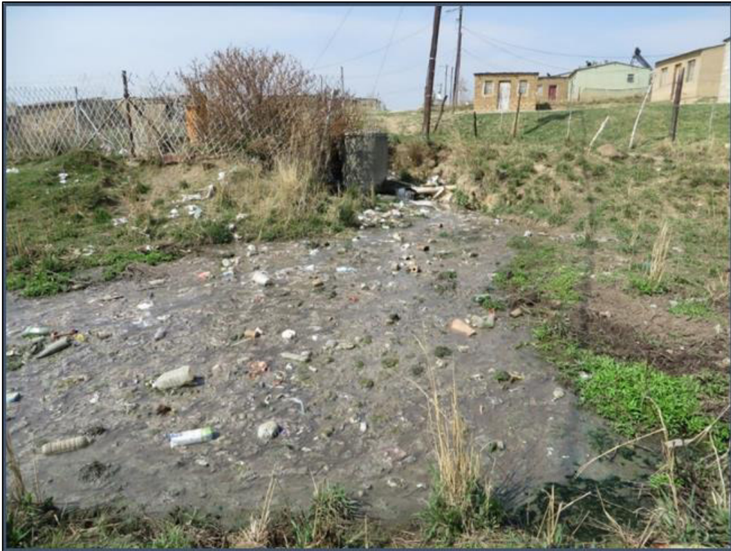
Plate 2: Site of a major and enduring leakage from a sewage line. The discharge is into a drainage line and wetland system.
