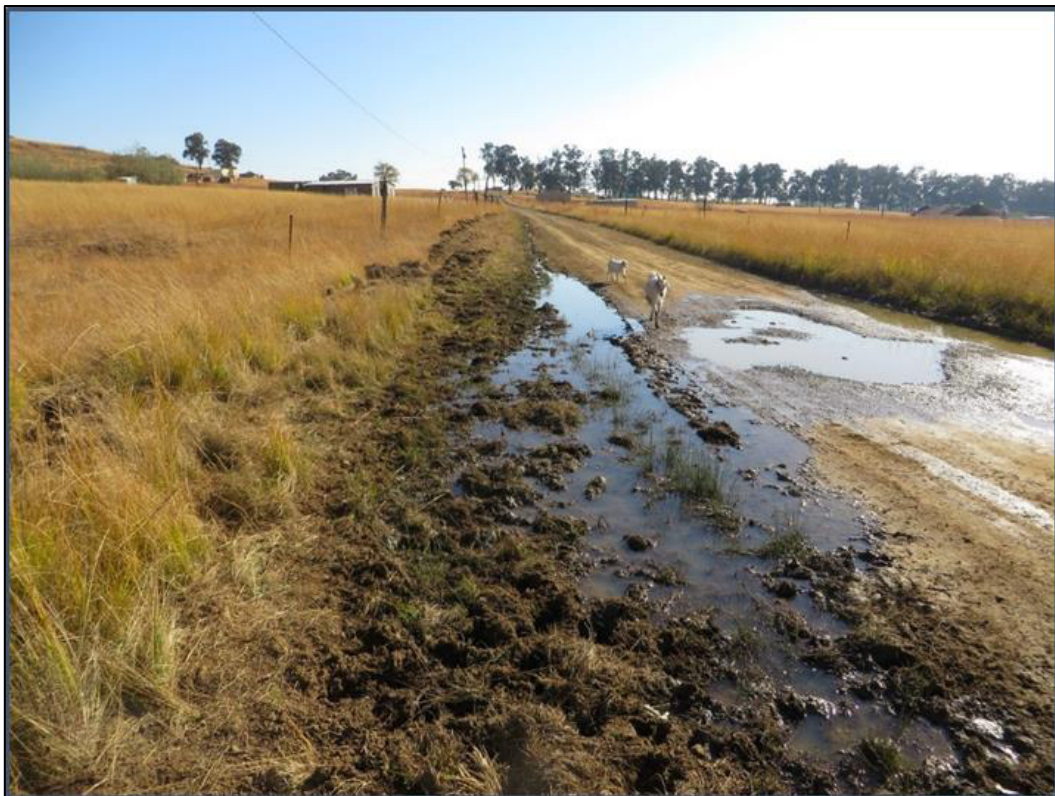
Plate 4: Water which has run down the road from a single tap which is located near the row of trees in the background. This leak supports a thriving wetland system and is also a watering point for livestock.
