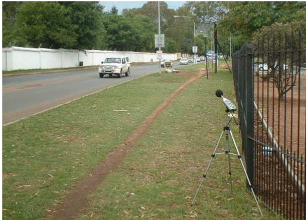
View Southwest along Club Street
