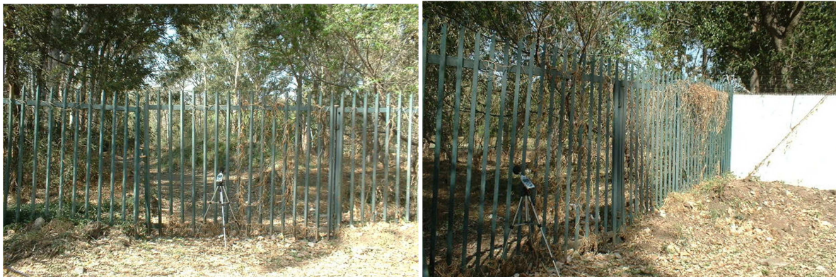
View into the site from Fairway street
