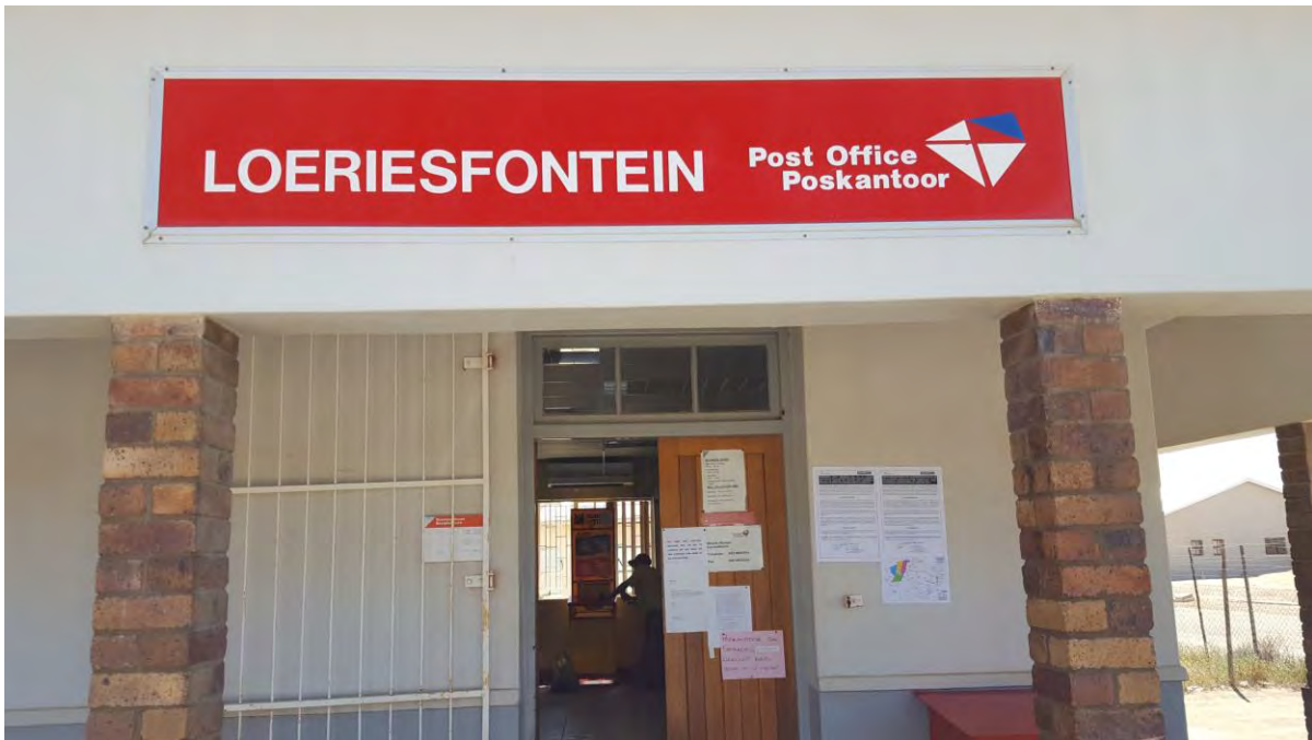
Figure 13: Post Office Entrance, Main Road, Loeriesfontein
