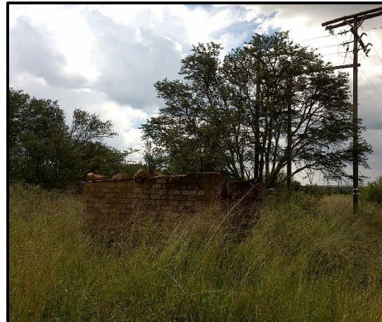
Figure 7-4. Electrical infrastructure leading to a pump house.
