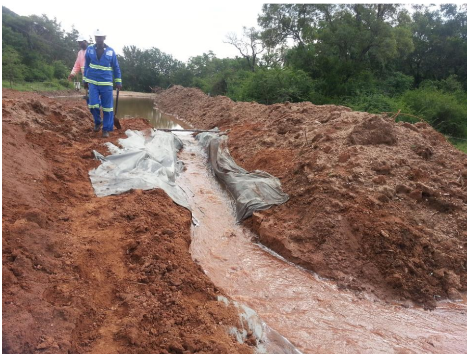
Photo 2. Lining of soil stockpiles prior to release of pooled storm water to ensure no loss of stockpile.
