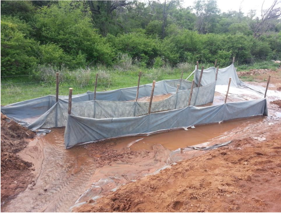
Photo 3. Silt fencing filtering sediment-laden water prior to water exiting servitude.
