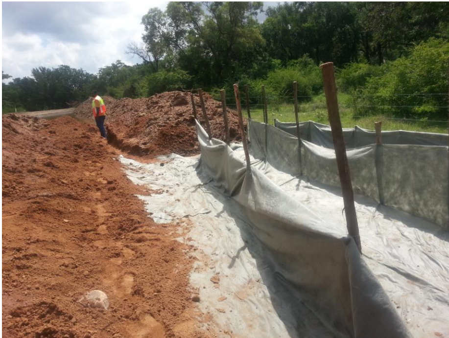
Photo 1. Installation of silt fence at discharge point.
