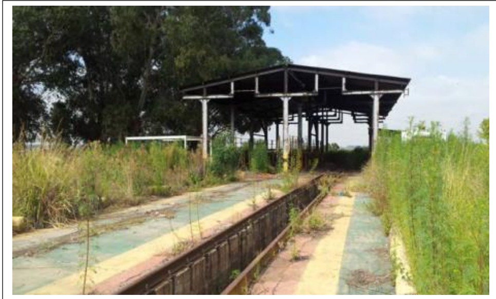
Figure 12- The rail way station along the railway line in close proximity of the Olifants River (Coetzee 2014).
