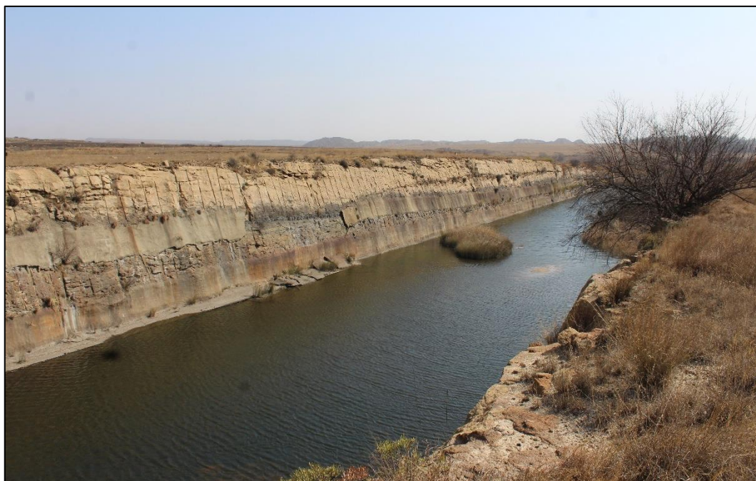
Figure 44: Significant channel and bed modification upstream of O3 (August 2018)
