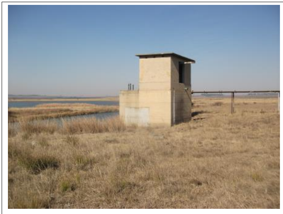
Figure 11- The pump station along the Olifants River which was used by the South African Railways.
