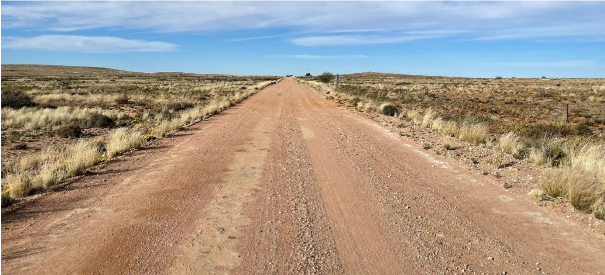
Figure 7.14 Existing Road DR2986 @ Km 148.11 – West Approaching
