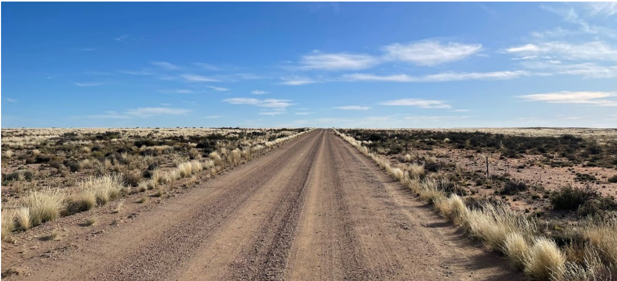
Figure 7.18 Existing Road DR2986 @ Km 142.80 – East Approaching
