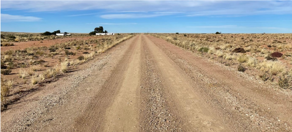
Figure 7.17 Existing Road DR2986 @ Km 146.82 – East Approaching
