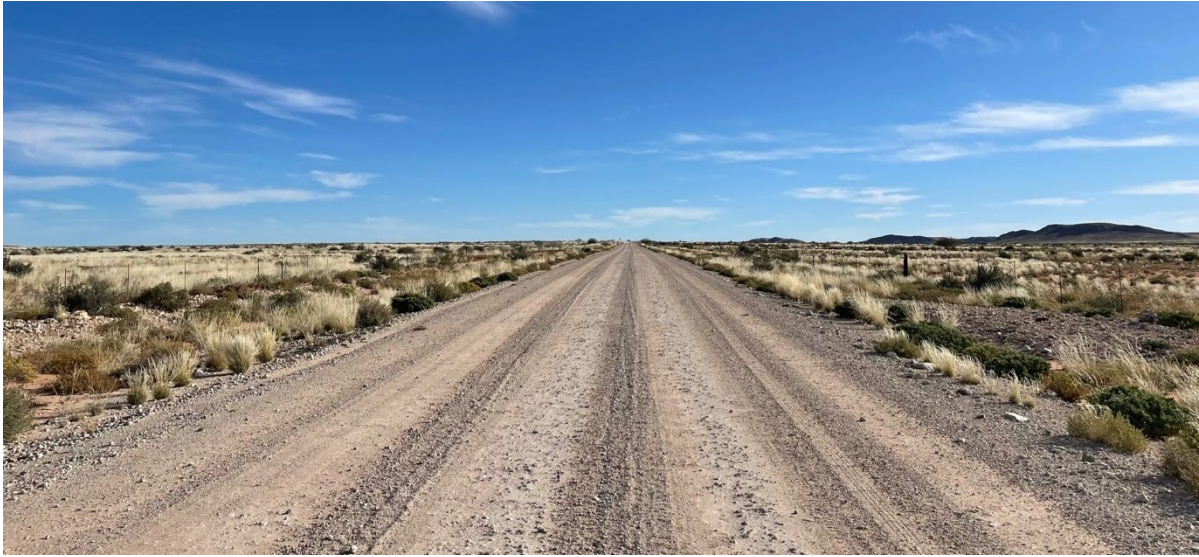
Figure 7.8 Existing Road DR2986 @ Km 153.99 – West Approaching
