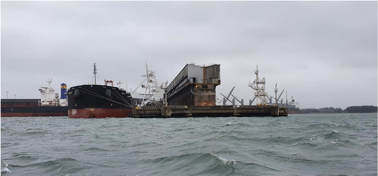
Figure 5-8 – Jetty to the north, from Location 7
