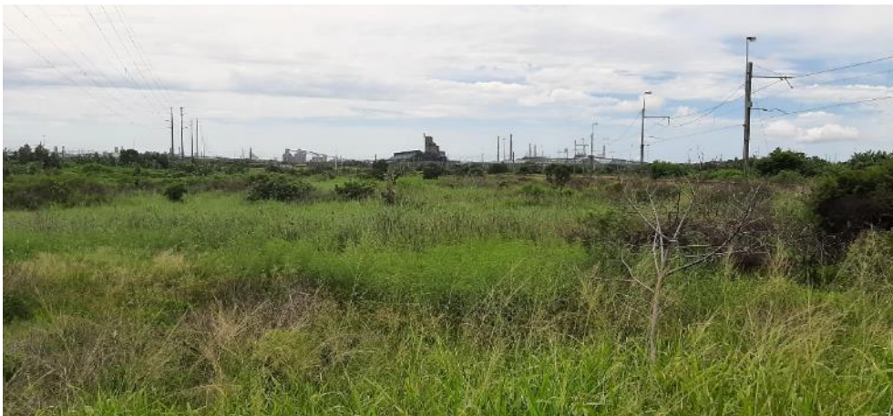
Plate 33. Overview of the upper middle portion of the existing powerline servitude (looking north east toward the Bayside Aluminium Smelter site)
