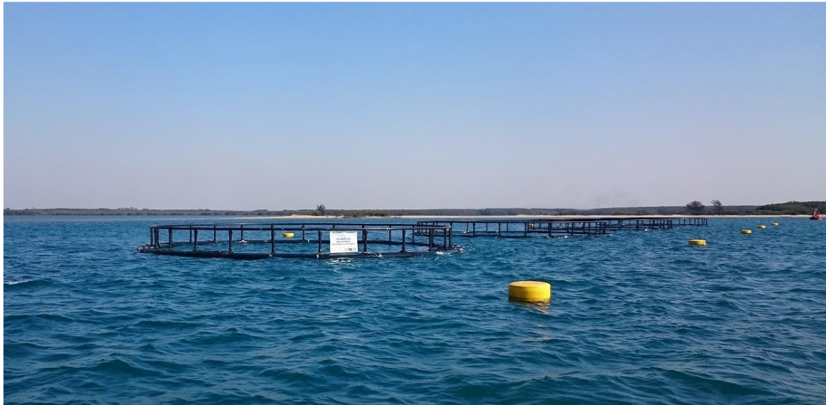
Figure 22: Four Fusion Marine Aquaflex cages installed in the port of Richards Bay as part of the DST SU KZN Aquaculture Development Project. (Source: Viljoen, 2019).
